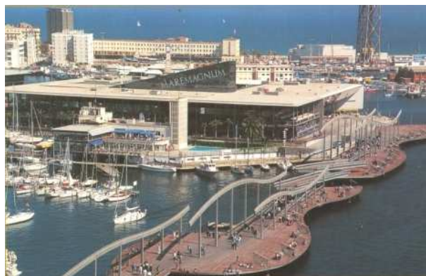
Figure 3. Maremagnum Shopping Centre (Barcelona, Spain)
